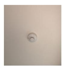
When there is a smoke-filled atmosphere, the smoke detector will be activated, and the alarm bells will ring throughout the building.
