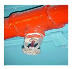
When there is fire and sufficient heat is generated, the sprinkler bulb or element will burst, and water will gush out to extinguish the fire. At the same time, the alarm will ring throughout the building thru the activation of the sprinkler flow switch.
