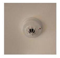
When there is a sufficient heat in the atmosphere, the heat detector will be activated, and the alarm bells will ring throughout the building.
