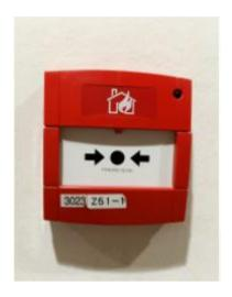
Smash the "Break-glass Call points with an object which will cause the release of the contact button hence ringing the alarm bells throughout the building.
