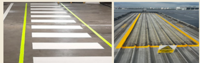
Left to Right: Reflective paint on driveway and demarcated hazard area with paint and warning signage
