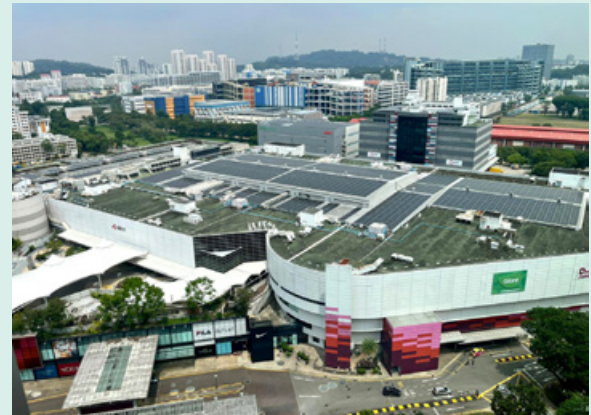
Solar panels on IMM Building's rooftop
